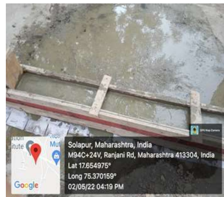
Fig.2 Casting of Beam
